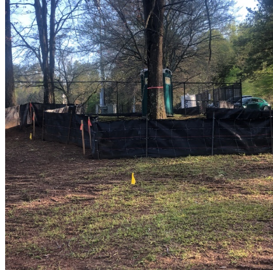
Silt Fence and Utility Locates
